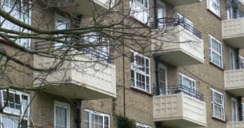
Glebe Court, showing the original building
