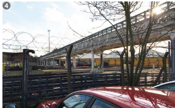
Figure 2-14 View of London Underground Depot
