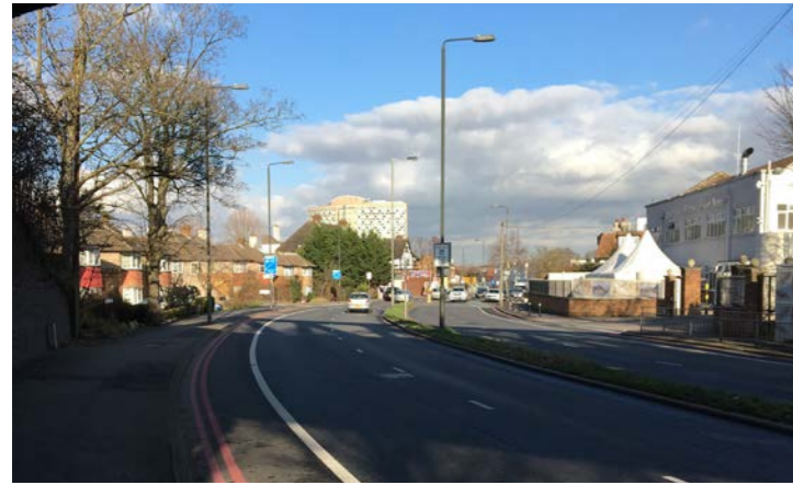
Figure 2-30 London Road approach towards Civic Centre
