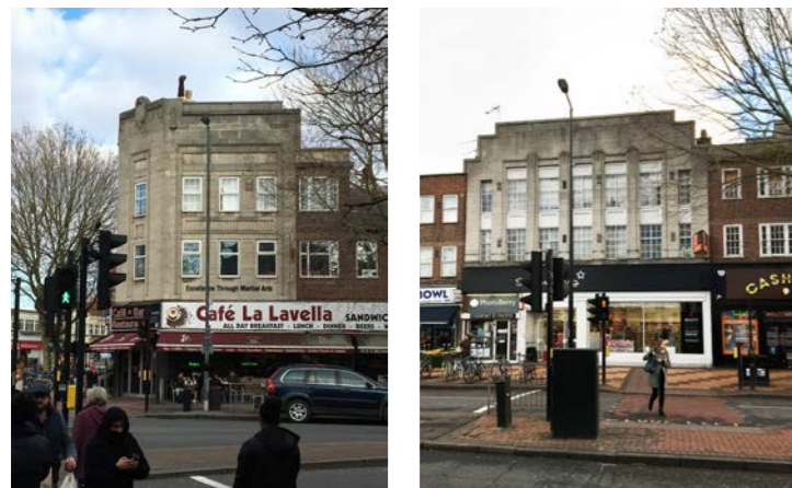
Figure 2-27 Occasional art deco stone feature buildings
