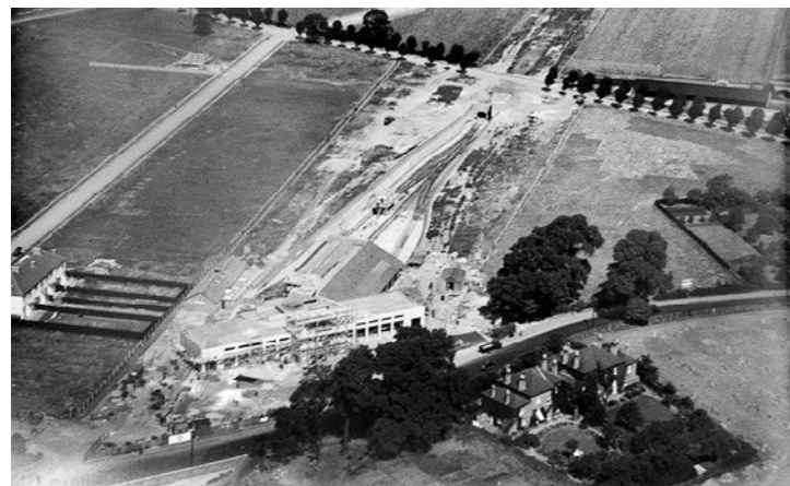
Figure 2-28 Construction of the underground station in 1929
