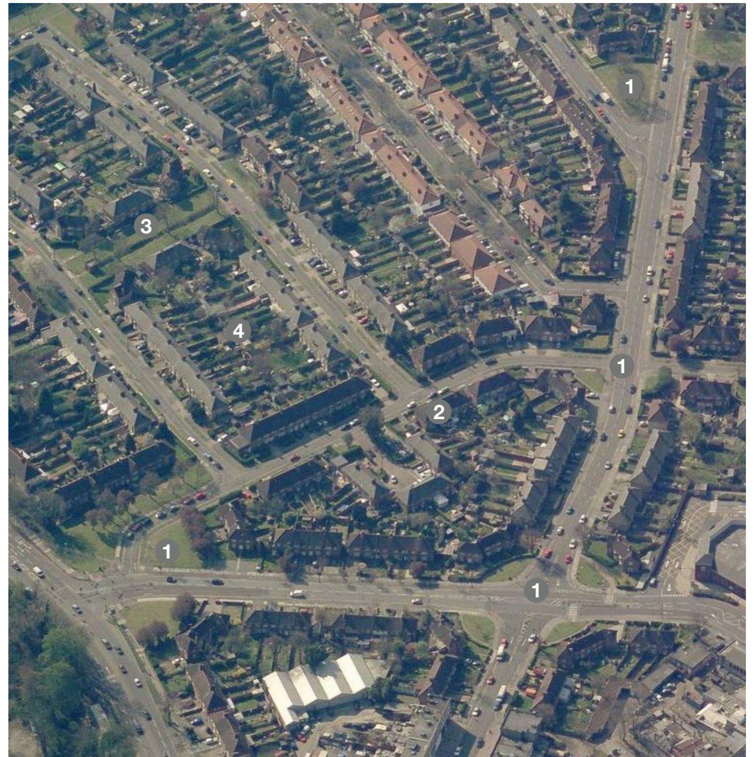
Figure 2-37 Aerial Photo of Abbotsbury Road
