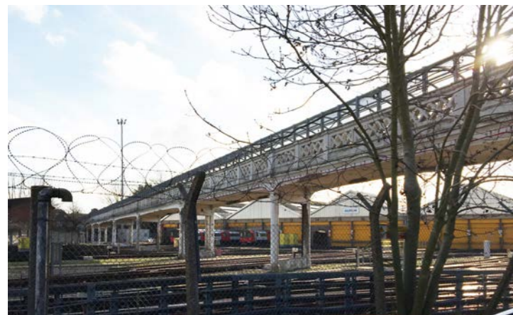
Figure 2-31 London Underground Depot
