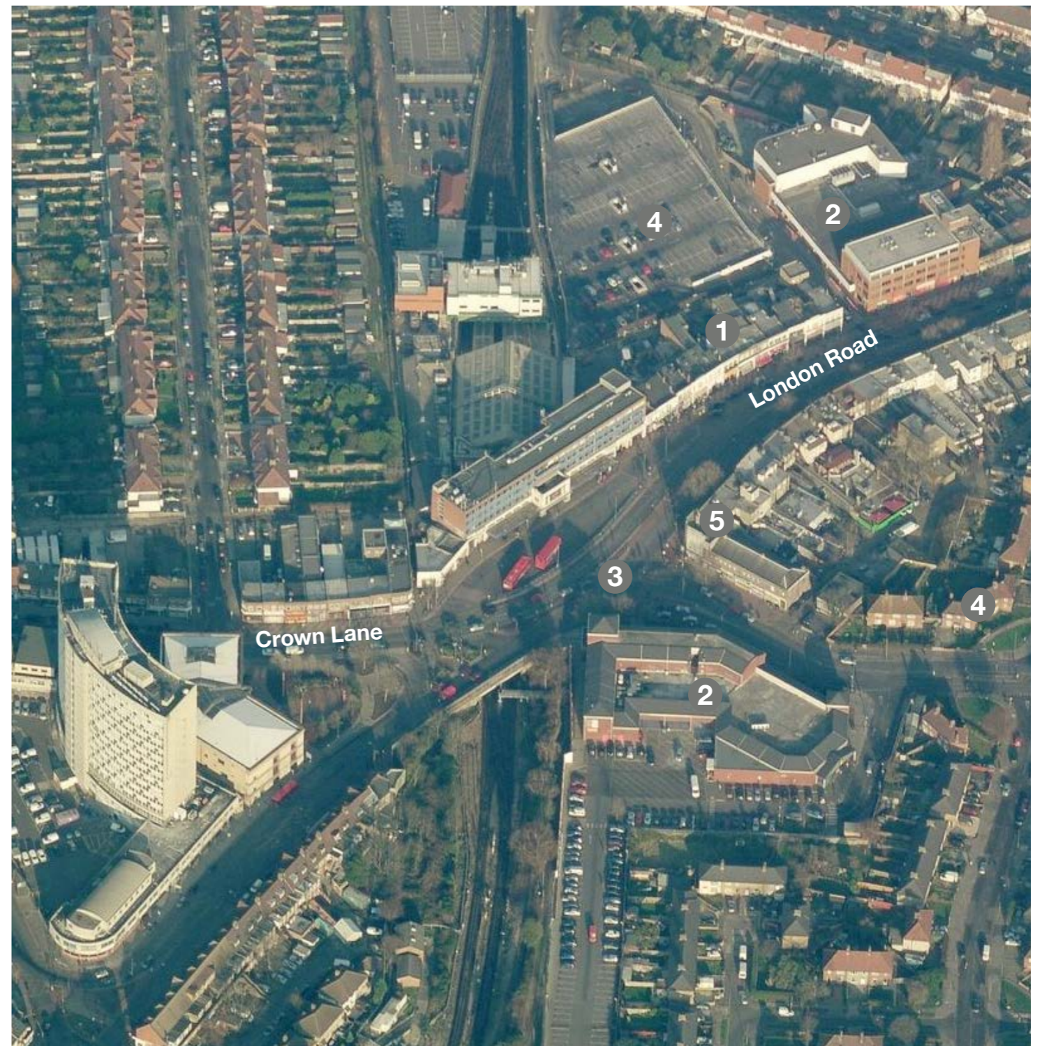
Figure 2-29 Aerial Photo of Crown Lane
