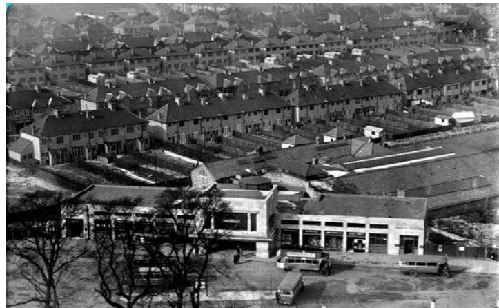
Figure 2-20 Housing constructed within 3 years of the station opening
