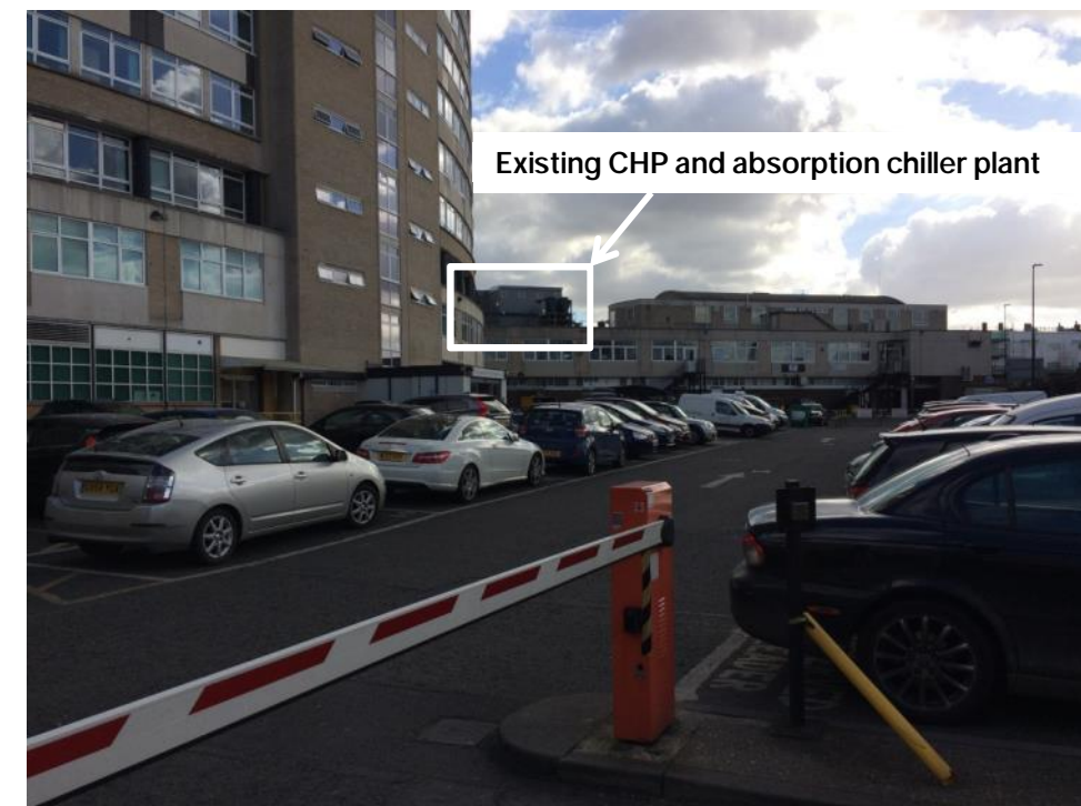
Figure 5-6: The rear car park of the Merton Civic Centre
