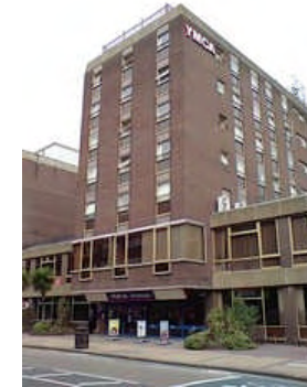
Figure 23: Example of high rise building – YMCA Building in Wimbledon TC
