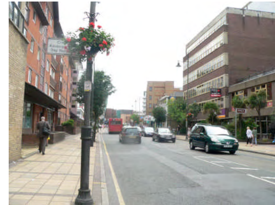
Figure 42: Tall building cluster along the eastern end of The Broadway
