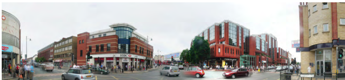
Figure 43: Tall building cluster around St Georges Road
