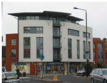
Figure 22: Example of mid-rise buildings in Wimbledon Village
