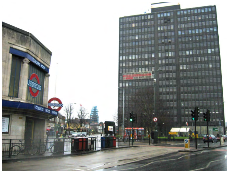
Figure 37: Brown and Root Tower Colliers Wood
