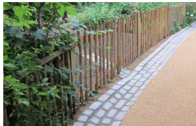
A granite sett channel collecting and conveying runoff at Holland Park, London.
