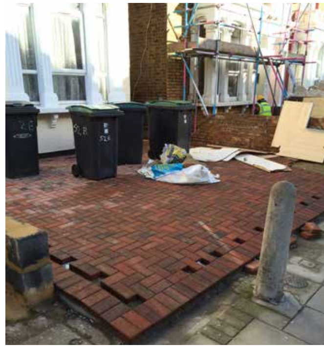
Paving over front gardens with impervious surfaces is increasingly common. This example could easily have been permeable block paved.
