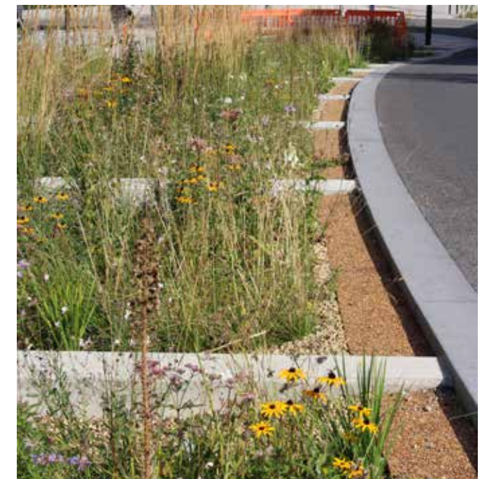
Attractive and wildlife friendly herbaceous planting by Sheffield City Council in a crushed stone bioretention substrate.
