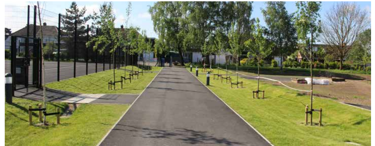
Linear swales alongside an entrance path at this infiltration SuDS project, Burlish Primary School.
