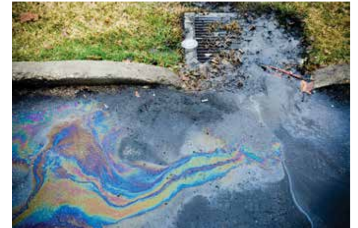
Typical diffuse urban pollution concentrated at a conventional gully.
