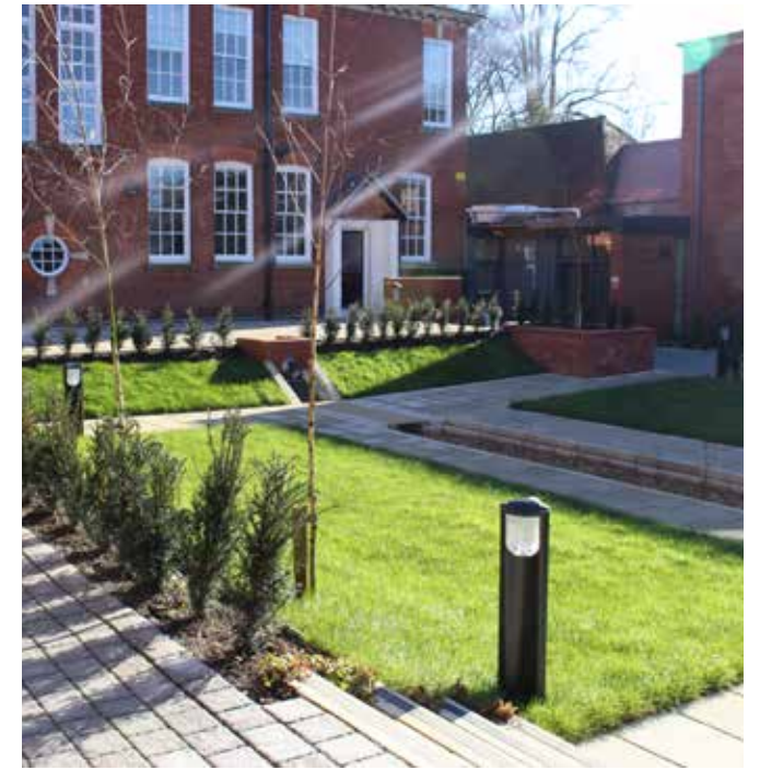
Parkside, Bromsgrove. Amenity grass shallow detention basin feature, integrated into site design, manages occasional extreme rainfall.
