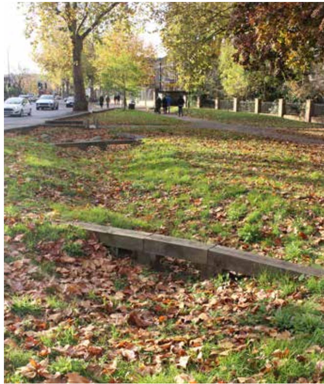
Rectory Gardens Rainpark, Hornsey. Forebays, swales and underdrained basins use SuDS turf (100-150mm) to filter runoff, with amenity grass for public use.
