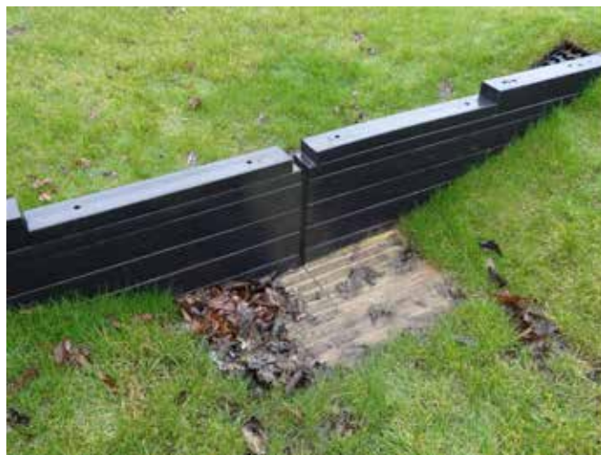
Flow controls in the landscape can make interesting features and help tell the story of how the system works. Although more prone to blockage, features such as this slot weir at Hollington School are very easy to unblock.
