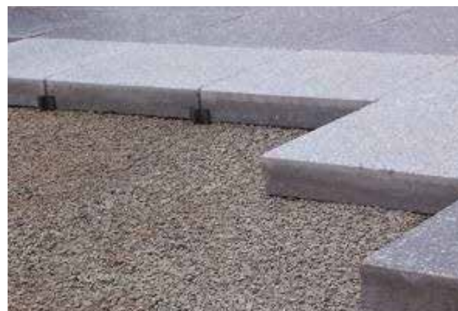
Plastic spacers are used to form open joints between standard slabs at Abbey Park Campus Leicester College, where all hard landscape areas, including the pedestrian entrance plaza to the building, are used for storage.
