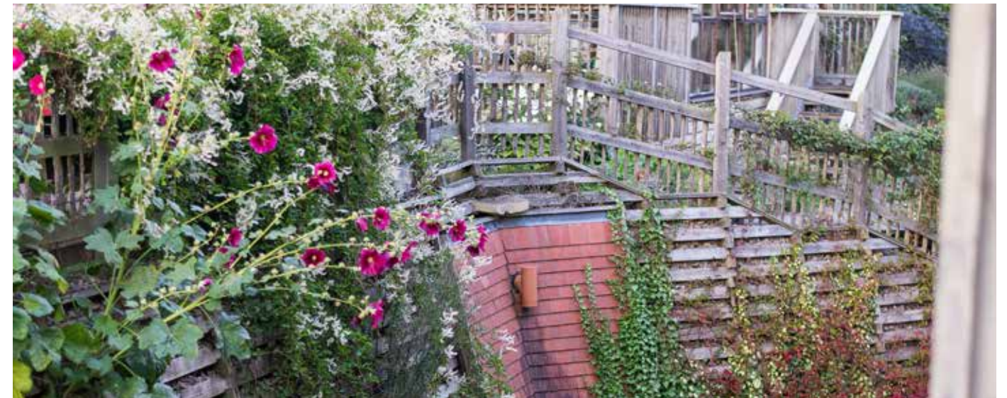
Springhill Cohousing, Stroud. Tile hung cascade conveys water through terracotta T-piece to lower level.
