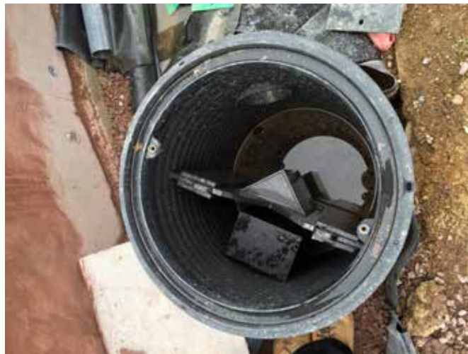
Orifice flow control chambers such as this one by Controflow are simple, reliable, cost-effective and easy to maintain.
