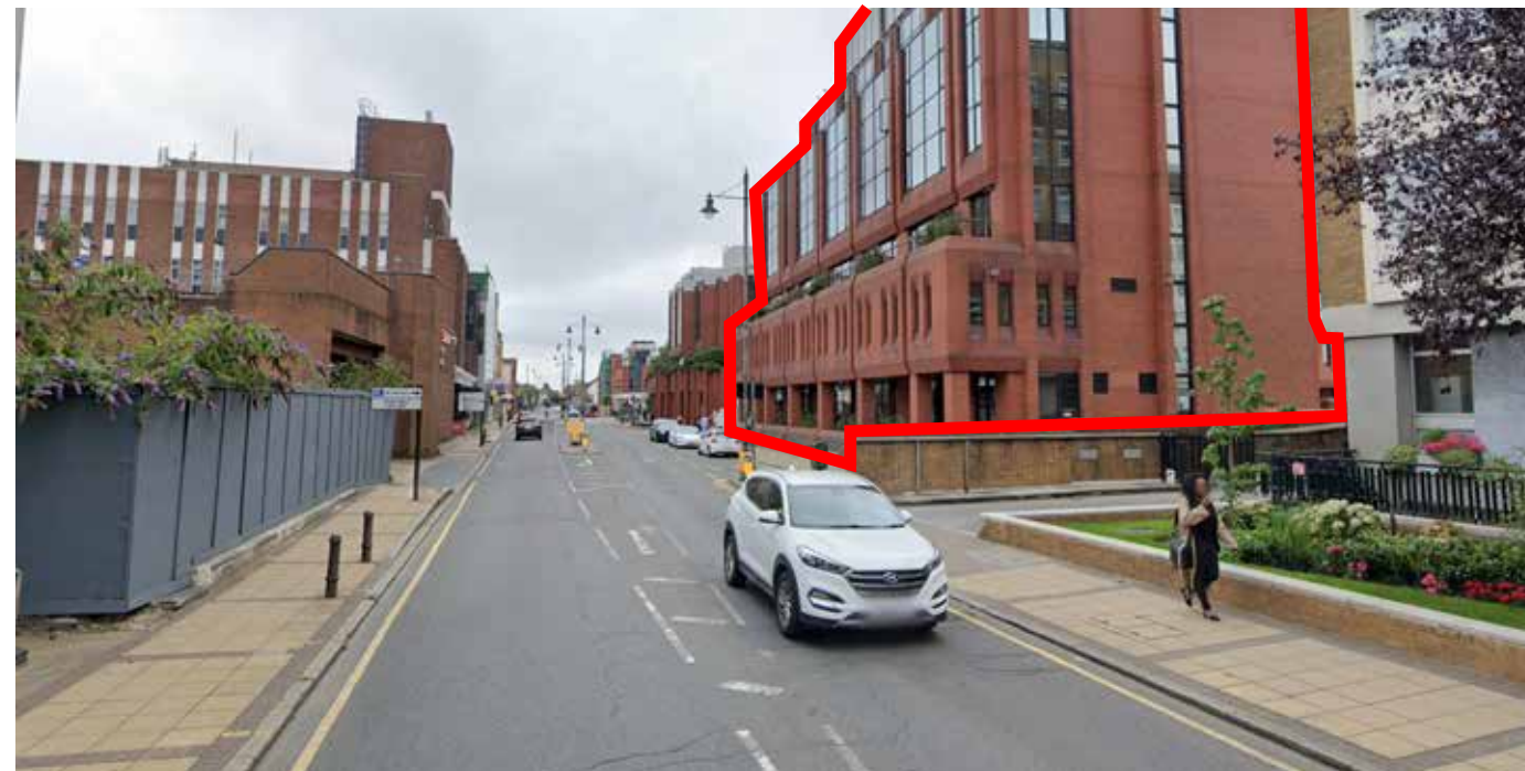
3. View from St Georges Road looking north
