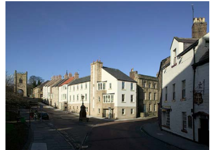
Flats are used to turn the corner of this urban block. Stepped bay windows and a large chimney stack to create a positive and interesting facade treatment on a prominent corner. Pottergate, Alnwick, Northumberland
