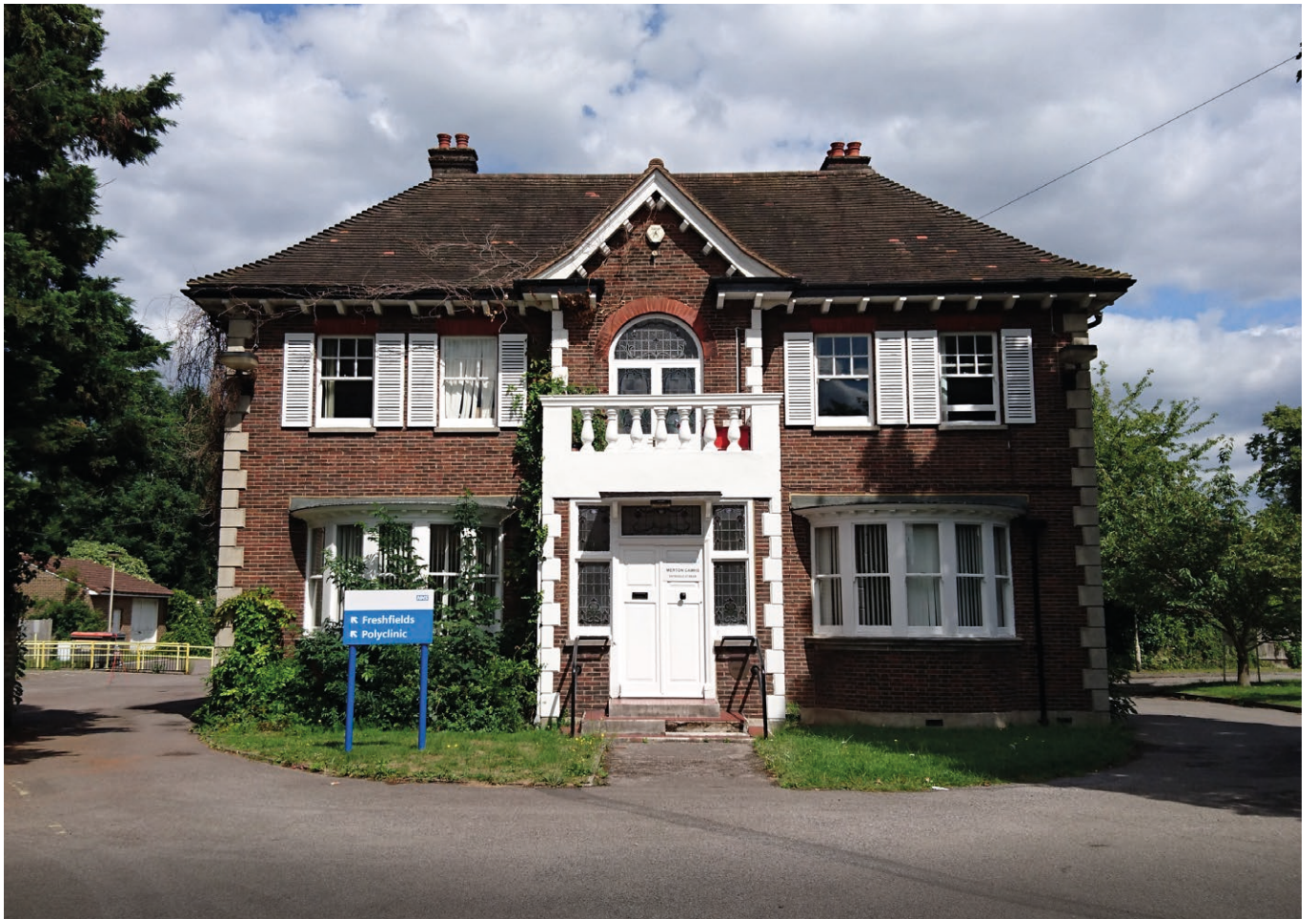
Fig.1 Front of site
