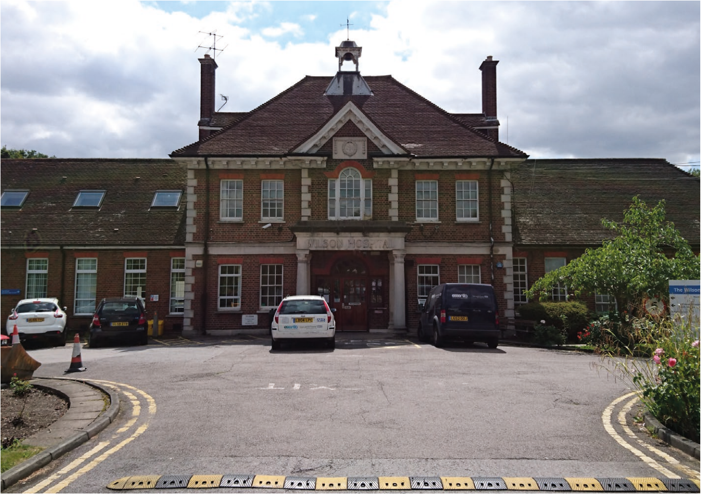
Fig.1 Front of site
