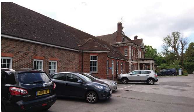
Fig.3 Existing hospital building looking west
