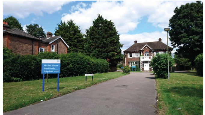
Fig.3 View of the entrance from Cricket Green
