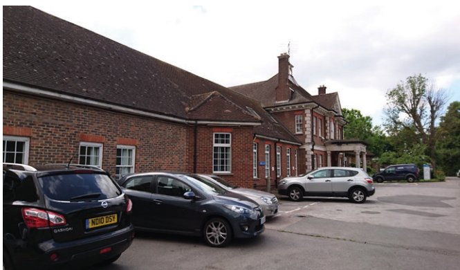
Fig.3 Existing hospital building looking west
